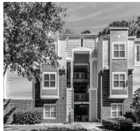
USV I – Hamilton Ridge Multifamily
